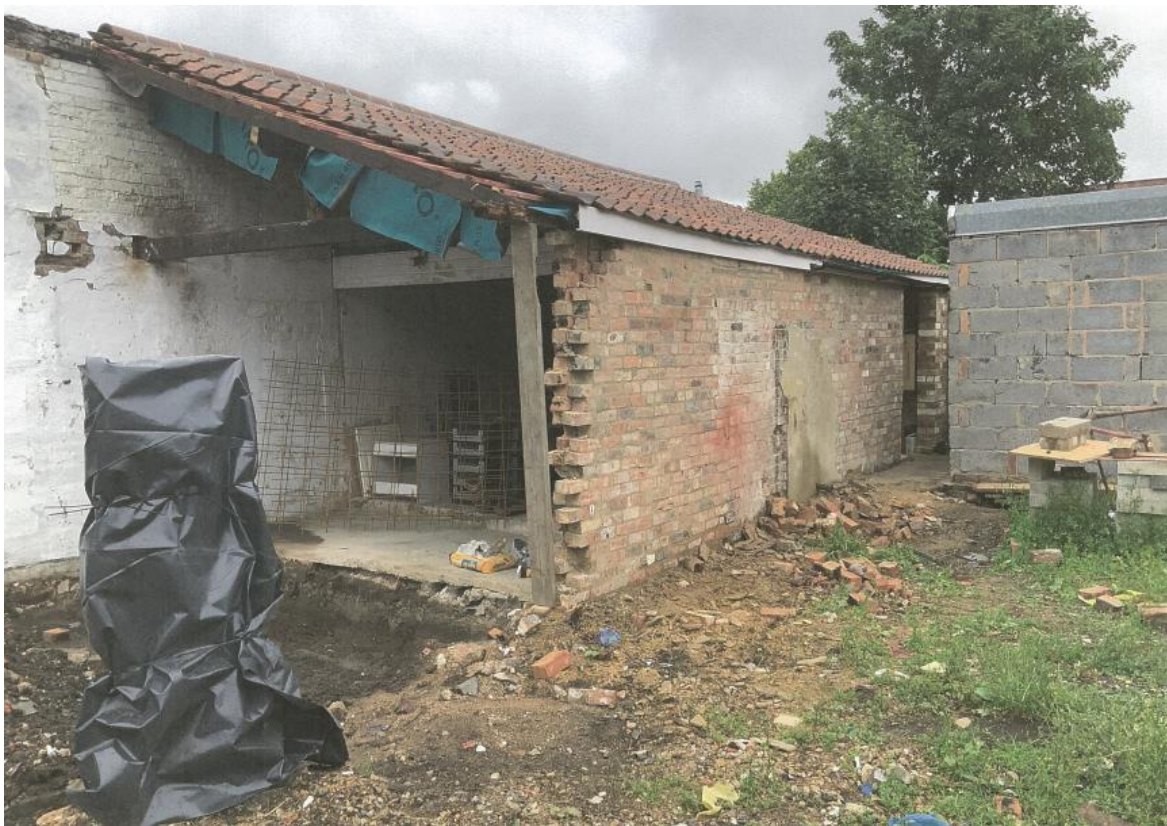
Outbuildings adjacent to east boundary, within ownership of 20 Saville Street
