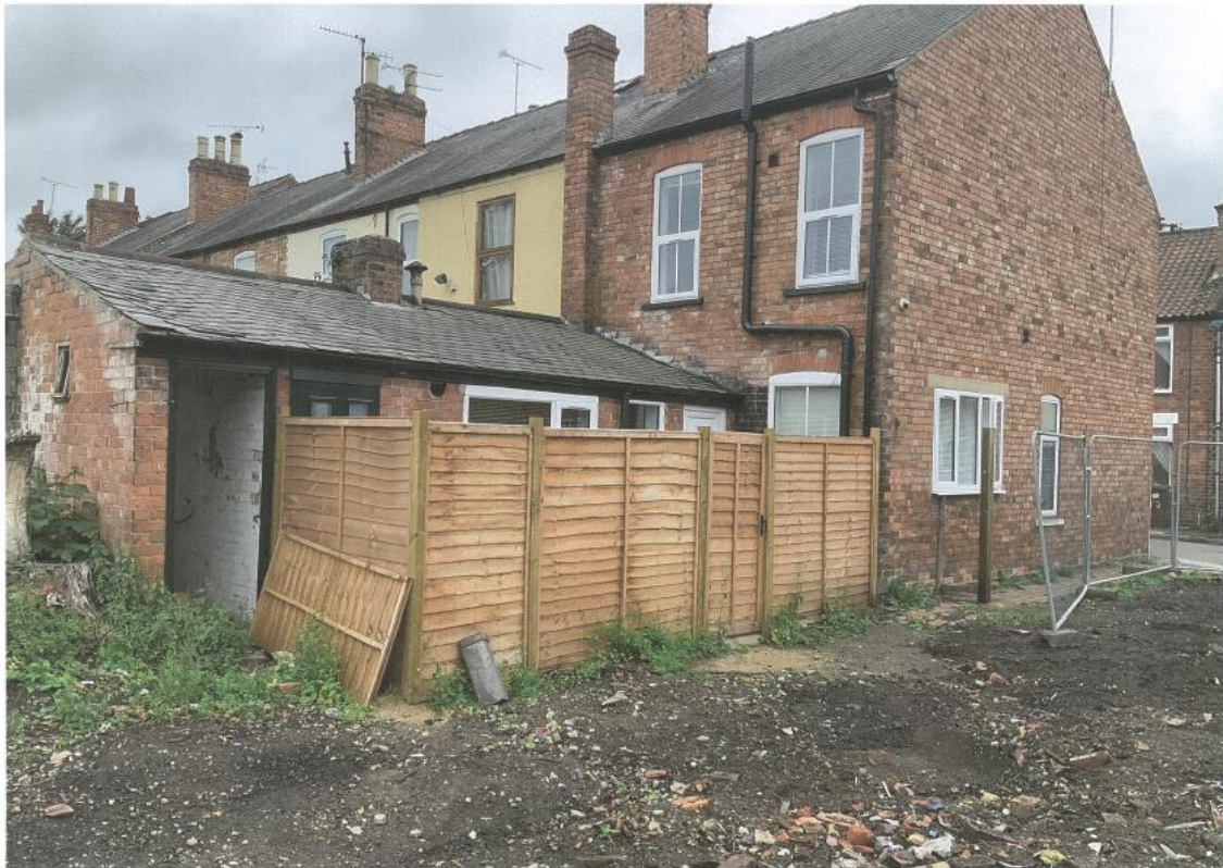
Side/rear elevation of 22 Saville Street (fence indicates boundary of no. 22's rear yard)
