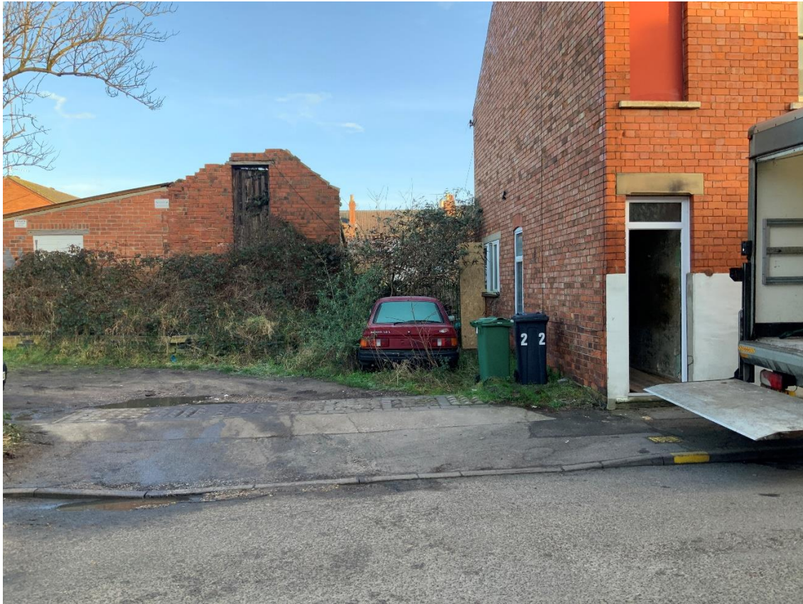
Existing access and outbuilding/garages with 22 Saville Street to the right
